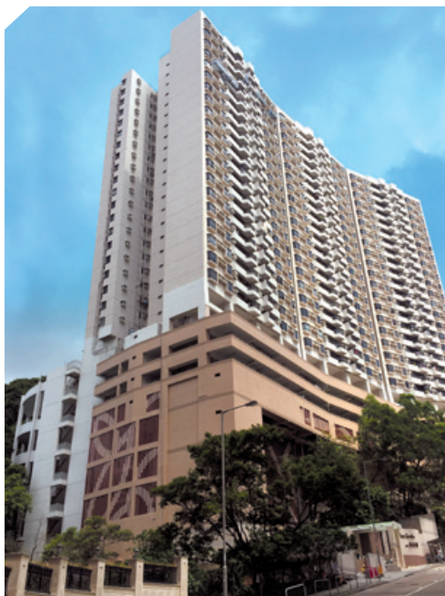
Exterior renovation of Flora Garden 慧景園之外牆裝修
